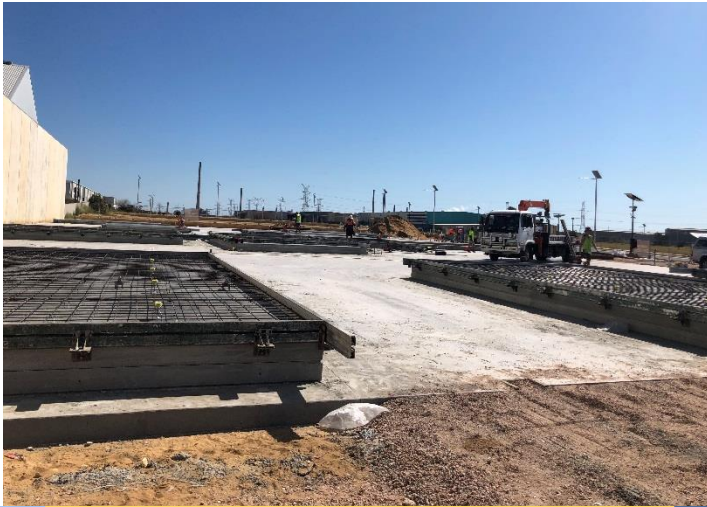
Progress of our new site – Tilt panels being poured and limestone wall under construction - exciting
